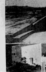
AUTO ENTRANCE ramp burrows inconspicuously into the desert as it leads down to a dual-purpose underground shelter and garage at the Operation Plumbat atomic tests in Nevada. Lower photo shows how the Alton blast crumbled part of the concrete retaining wall but failed to block the entrance. To the right of the crumbled wall is the entrance, closed by a 108-in. four-foot-thick reinforced concrete blast door (inset), which was undamaged. (OTTO LOWERY/STANLEY LEB PHOTO)
