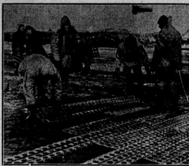
Bureau of Public Relations, U. S. War Department AVIATION ENGINEERS IN THE ARCTIC —A vital link in the chain of air bases built by U. S. Aviation Engineers is this landing field somewhere in the Aleutians. The field having been cleared, graded and rolled, portable steel landing plank is laid to complete the intricate system of runway and taxiways from which our aircraft will carry the war to the enemy.
